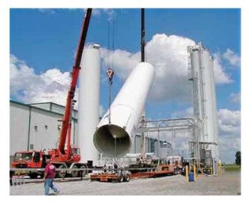
the book, *Structural Analysis of Shells* by Baker, Kovalevsky, and Rish.<sup>2</sup> The tank product area should be designed according to Janssen's formulas for cylindrical bins, which are used to calculate the vertical and lateral pressures in a silo by the bulk solid material.
