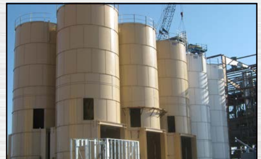
21' x 56' - 500 ton truck load-out silos (6 & 8 pack configurations)
