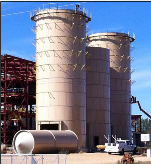
Standard 24' x 80' each storing 1,000 tons of frac sand.
