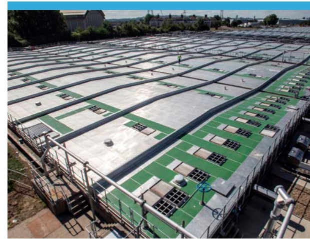
» Beckton Sewage Treatment Works United Kingdom – Approximately 600,000 sq. ft.
