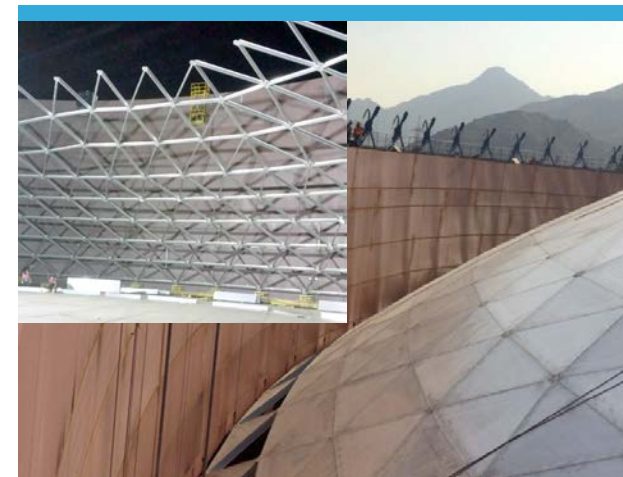
» National Water Company Makkah, Saudi Arabia – 361' Diameter
