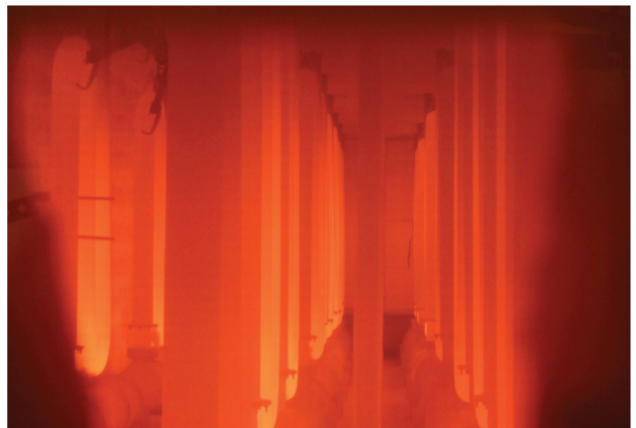
Figure 1 – Environmentally controlled coating application booth with positive pressure environment.
