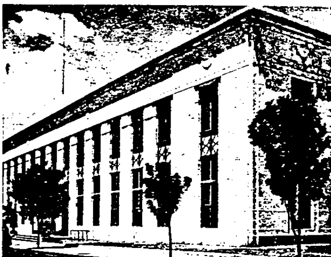
Figure 15—U. S. Government building at Key West, Florida, erected 1932, using windows of extruded aluminum alloy (alloy 43). The seaside conditions prevailing at Key West have had little effect on these unpainted aluminum windows. This photograph, taken in 1944, illustrates the non-staining characteristics of aluminum alloys.
