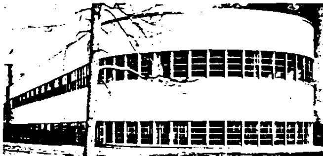
Figure 13—Laboratory of Federal Telephone and Radio Corp. Nutley, New Jersey. Easy to erect insulated panels of aluminum alloy 3S form the weathering surface of this unit erected in 1945 and for units subsequently added. Large numbers of windows of extruded aluminum alloy 635 were also employed. In this non-industrialized environment the bare aluminum alloy surfaces will slowly weather to acquire a uniform light gray patina.
